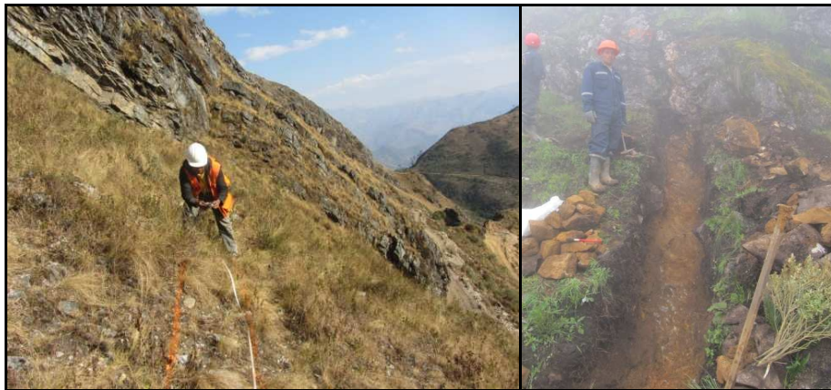
FIGURE 9-14: EXAMPLE OF A TYPICAL SURFACE TRENCH
