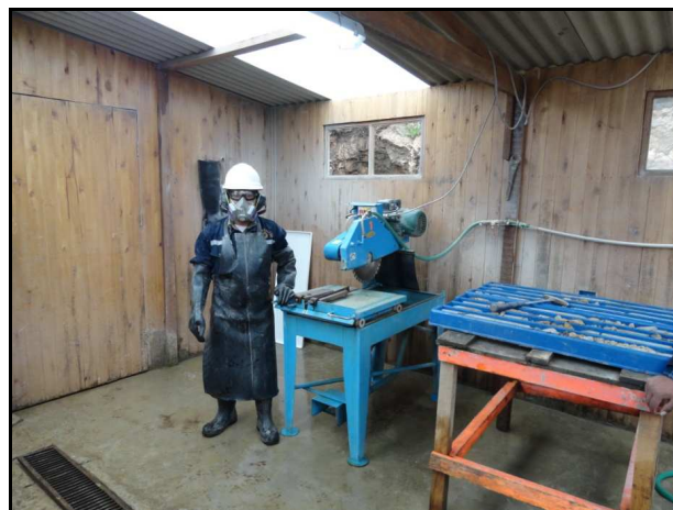
FIGURE 11-9: CORE SAWING SHACK
