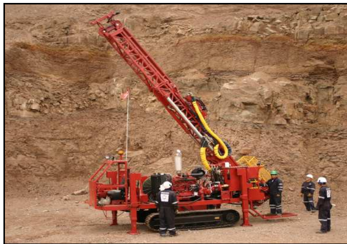
FIGURE 10-4: SANDVIK DE-710 DRILL RIG
