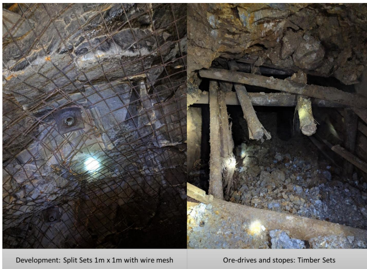
Figure 16.7 Current Ground Support, Igor Mine
